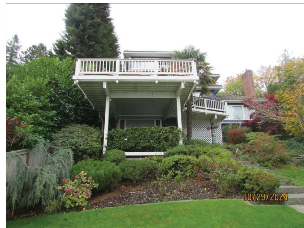
EAST SIDE OF THE DECK
